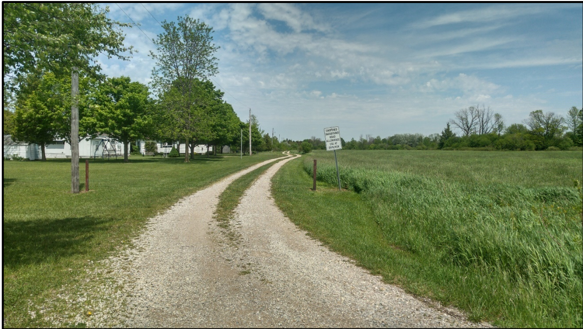
Image 7: Huron Street South from Intersection with Ashfield Street (looking north)
