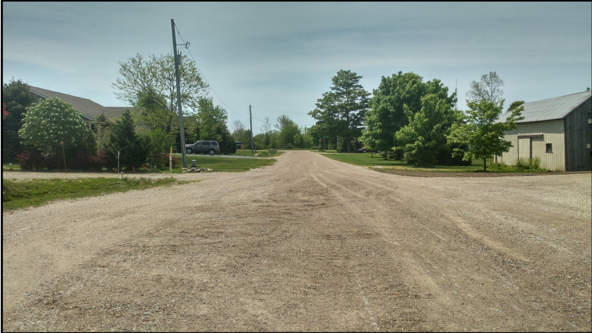
Image 21: Sydenham Street North of Ashfield Street (looking south)
