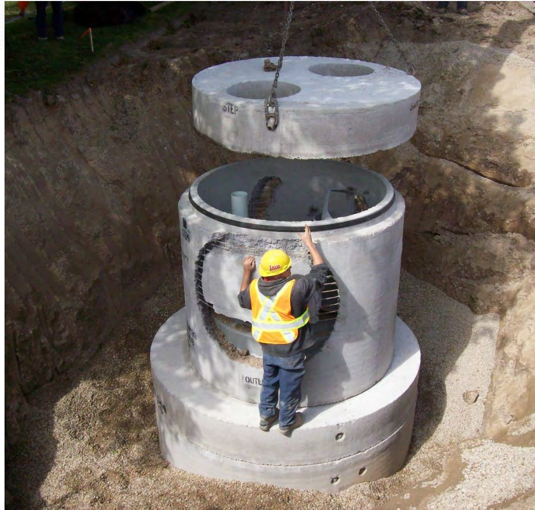
Stormceptor installed on London Road
